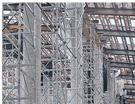
With large loads, the ST 100 Pivoting Head Spindle can also accommodate steel walers and other steel profiles.
