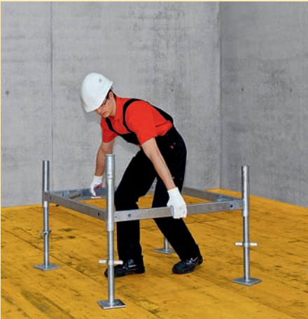
Set up the basic frame – adjust base spindles to required height and level accordingly.
