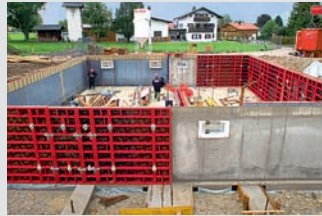
Wall Formwork
