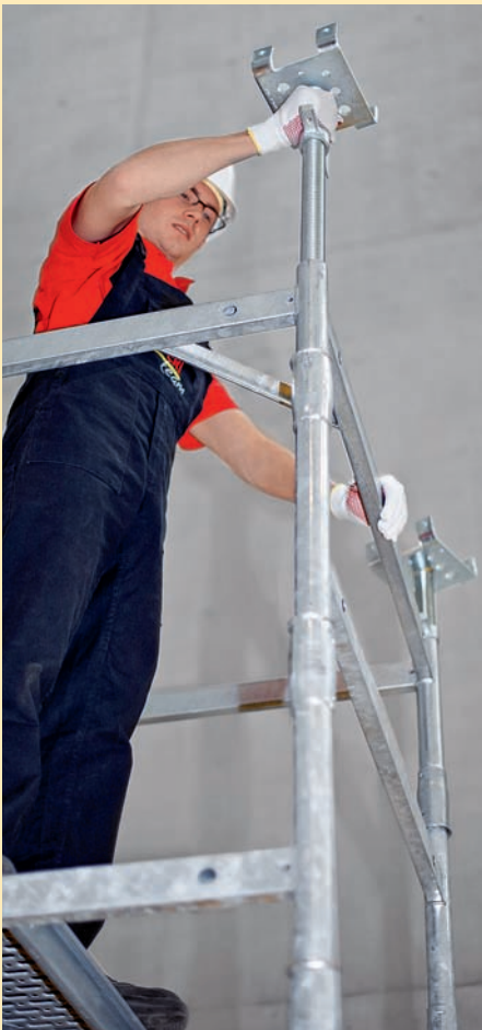
Adjust the head spindles to the required size and insert.
