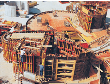
Through the combination of different formwork systems, the complicated ground plan of this office building could also be cost-effectively formed.
