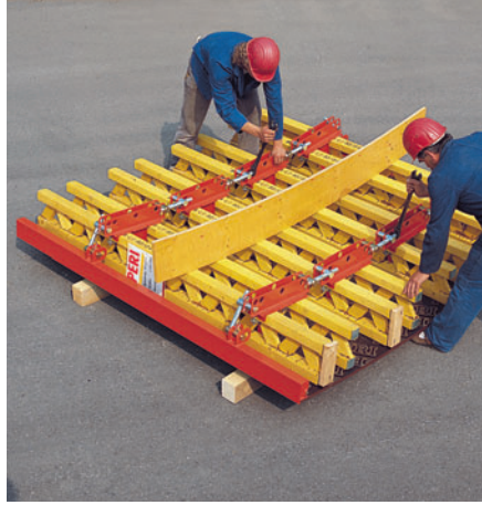
Checking the required curvatures is carried out by placing the radius template on the formwork girders.
