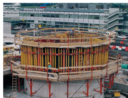
Spindle core and parapet of a spiral ramp for a multi-storey car park. Simple radii adjustment with the self-cleaning hexagonal spindle.
