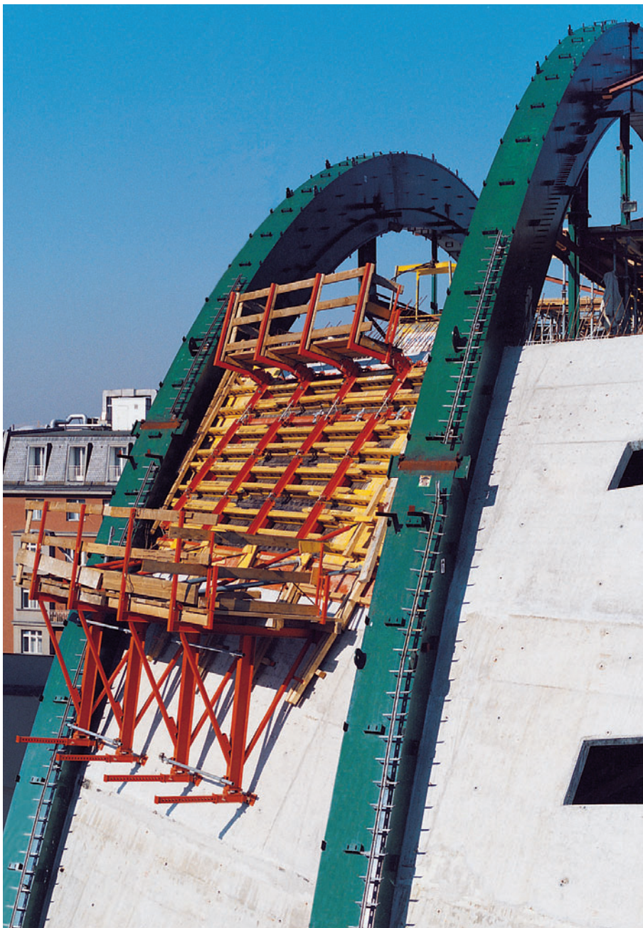
“Horizontally” positioned RUNDFLEX for the forming of an arched slab for a culture centre in Berlin.
