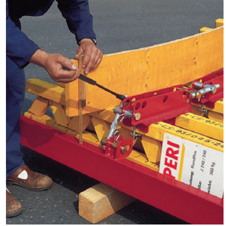
The "combi" ratchet spanner is used on the Adjustable Spindle 210 to adjust the edge profiles.
