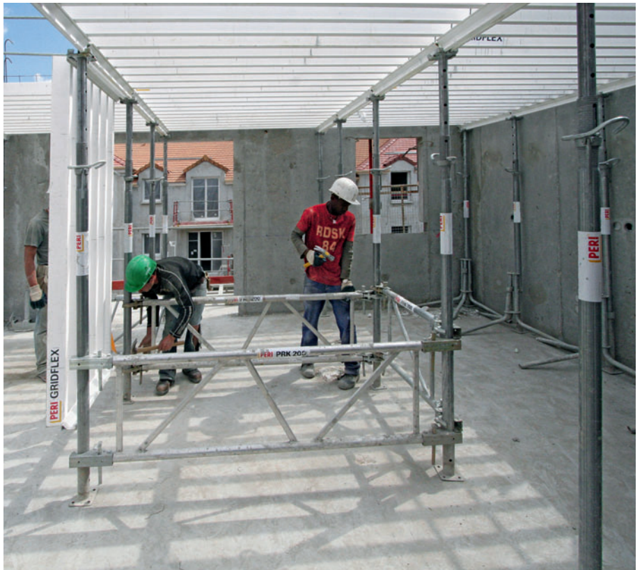
The PERI Ergo tripod and the PERI PRK frame are used as assembly aids.
